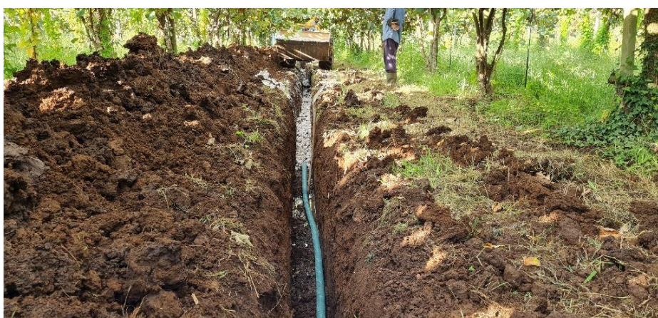
Figure 2. Excavations for the setting-up of the water drainage plant.
